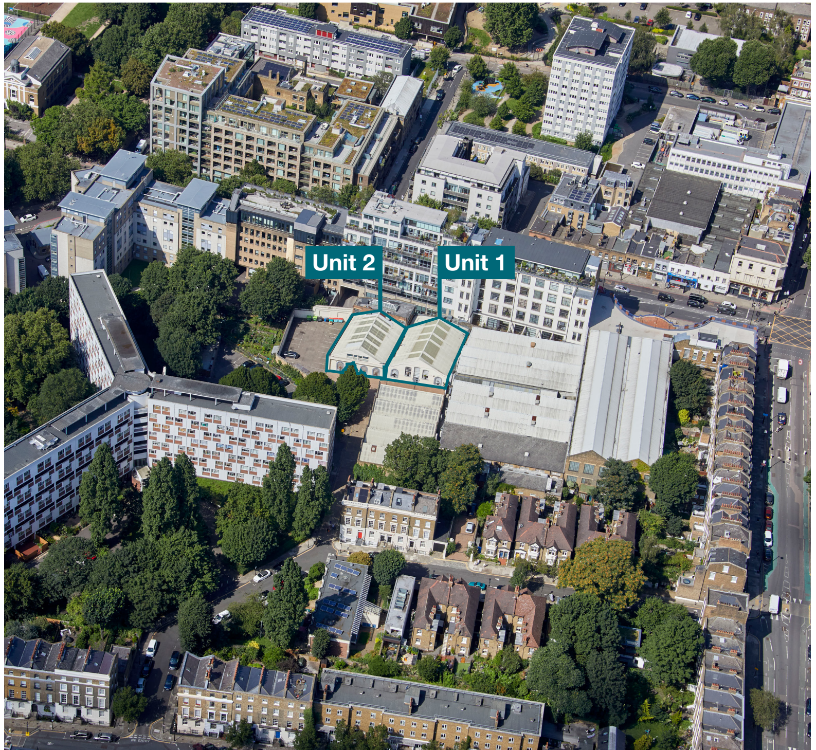
Holford Yard comprises of brick-built, period warehouse buildings with steel truss roofs. The two newly refurbished, light industrial units are situated within a gated compound with loading and parking.
