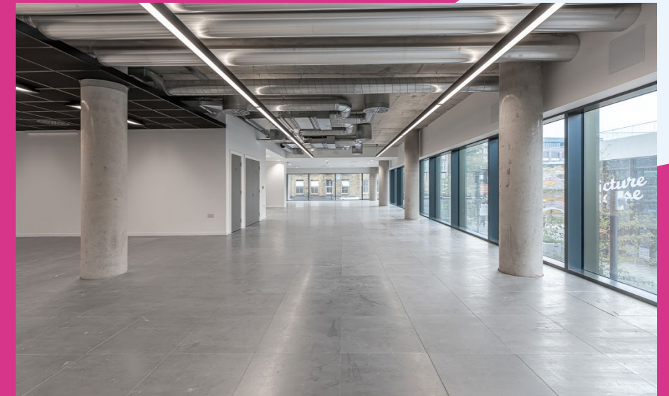
Current CAT A fit-out of Carriage House
